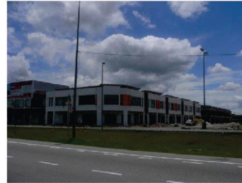
(a) Under construction commercial shops
